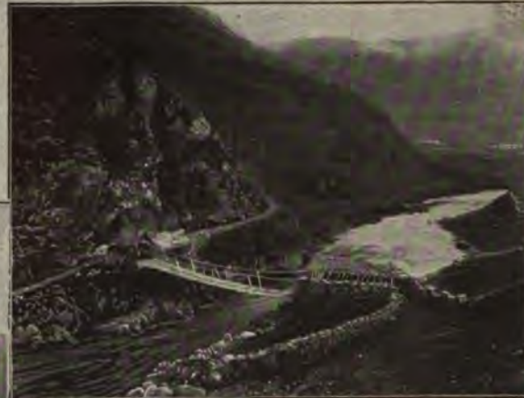
A wire bridge over a mountain stream on the eastern slopes of the Andes in Peru.
